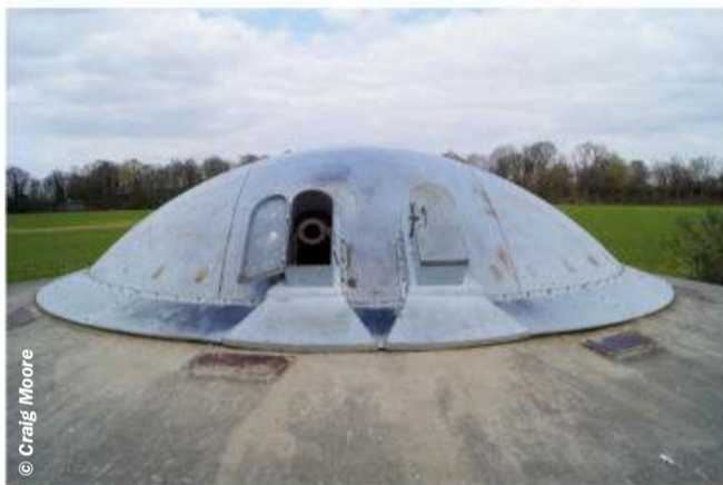
On the Eben-Emael fortress roof there was a revolving heavily armoured cupola with two 120 artillery howitzers
